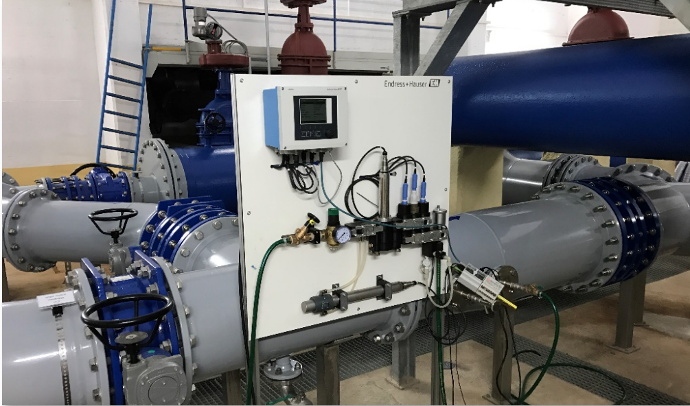
Water quality measuring station: sensor problems
